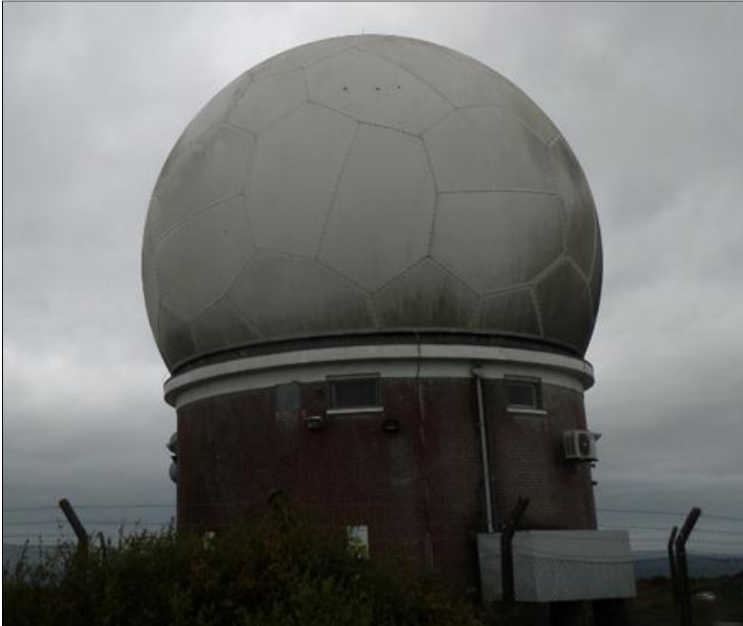
Figure 10. Woodcock Hill Radar Station
